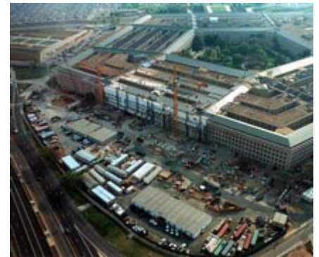
Rebuilding of the façade damaged in the 9-11 attacks.
